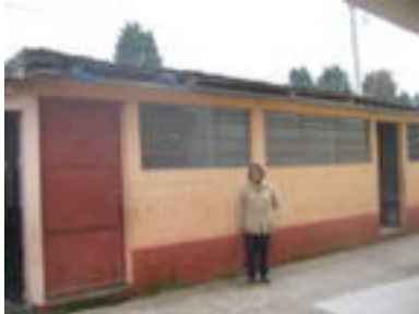
Classrooms before construction
