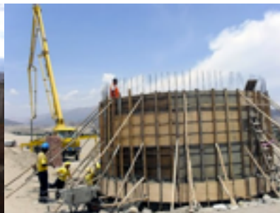
Building the water treatment facility
