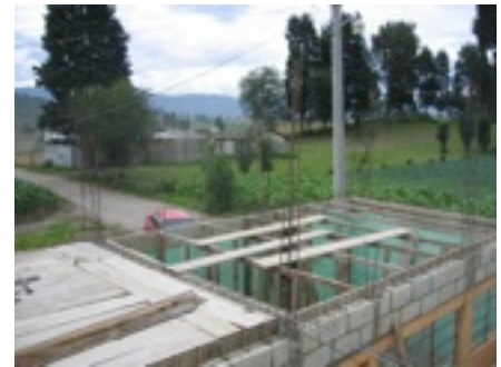
Wooden supports for new ceiling
