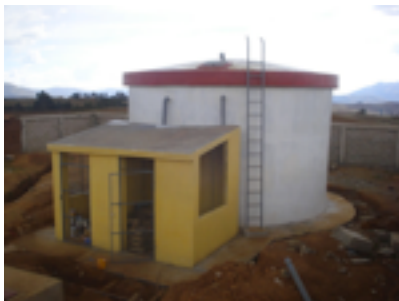
The complete water treatment facility
