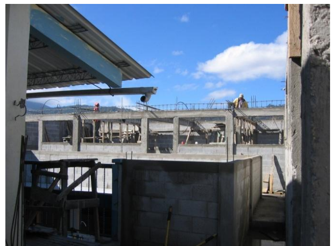
Work near completion on 2 nd story of Tierra Colorado school
